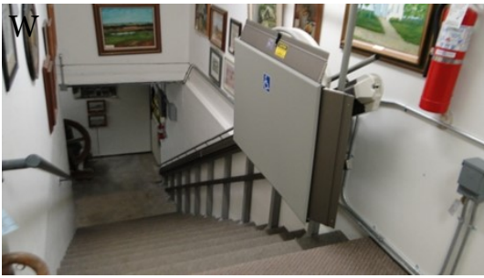
New lift to our basement is installed
