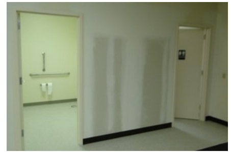
2 new handicapped unisex restrooms
