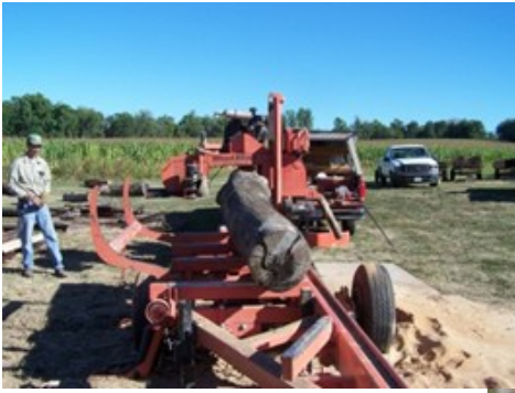
Milling replacement logs at Lynn Hommer's farm with portable saw mill.
