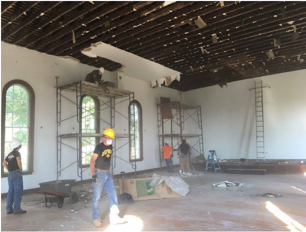
September 24th work day to remove ceiling due to mold
