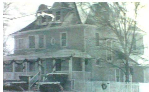
House Morrison built. Larry McConnell lives here now.
